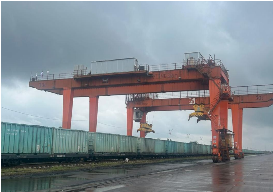
Figure 1. RMKE's Crane Facilities
