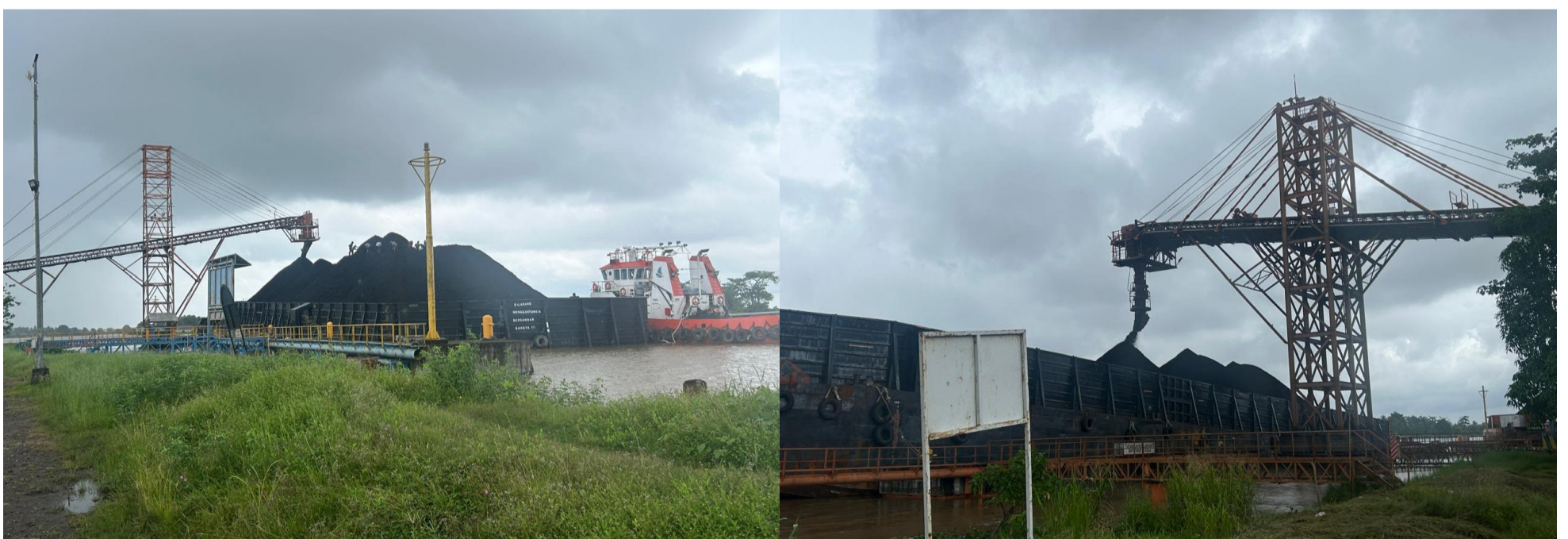
Figure 5. RMKE's Dual Jetty Infrastructure
